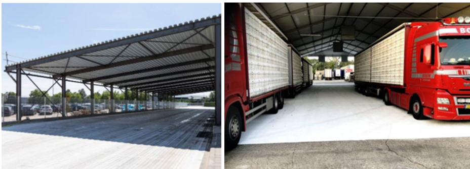
White asphalt to reduce heat absorption from the roadway into the livestock trucks
